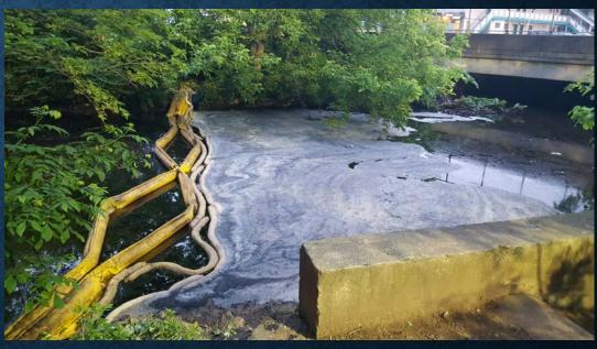
THE RESPONSIBLE PARTY WAS UNABLE TO ENGAGE A CONTRACTOR SO STATE FUNDS (\$160,000) WERE USED, THE DEPARTMENT'S CONTRACTOR WAS DEPLOYED TO THE SCENE 4 VAC TRUCKS WERE USED TO RECOVER POOLED GASOLINE ON THE ROADWAY AND IN WEST BROOK. SORBENT AND HARD CONTAINMENT BOOM WERE DEPLOYED IN THE BROOK.
