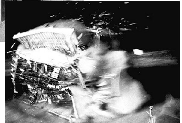
Thermal pulse ignites paint and wood
