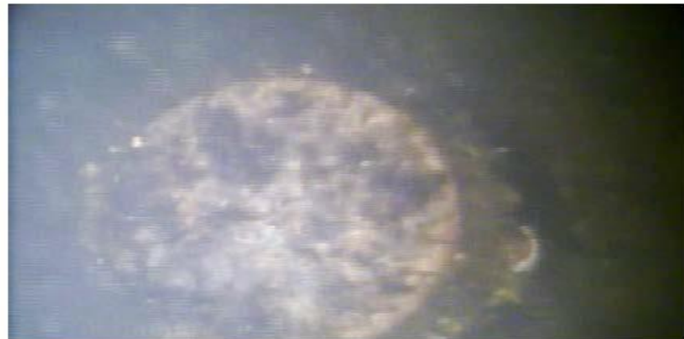
Capped Piping on top of Hatch Cover
