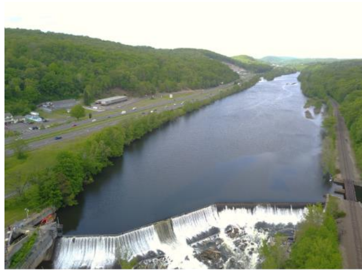
Kinneytown Dam looking upriver. DV-01b to right. Fish Ladder and site of CB-02b on left.
