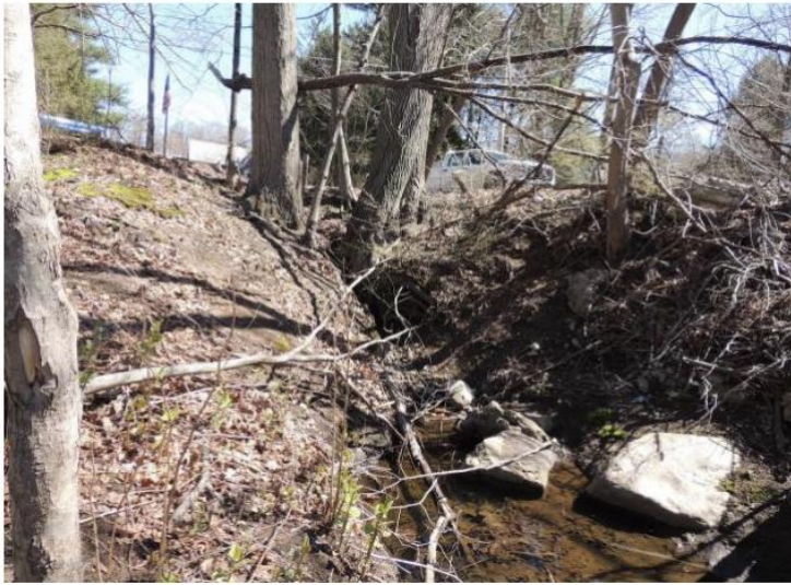
Culvert along east bank of river along Platts Mill Rd.
