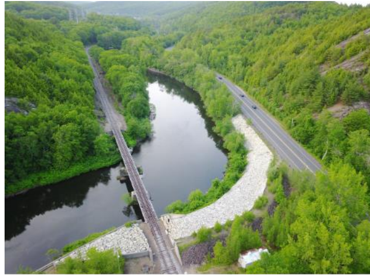
Site of DV-01 looking upriver.
