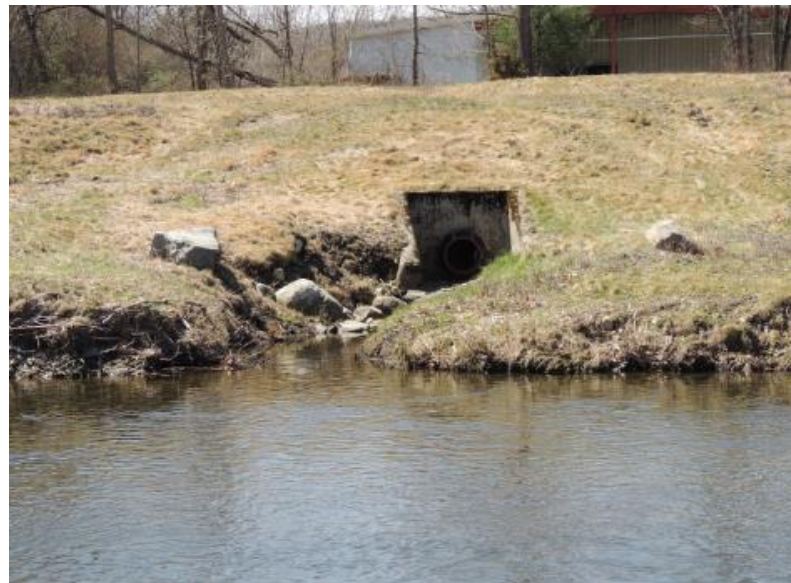
Culvert on west bank of Naugatuck River behind 699 S. Main St.
