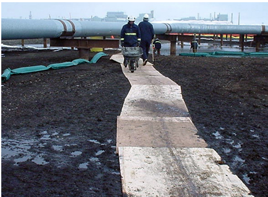
Figure 13. Using plywood to avoid trampling
