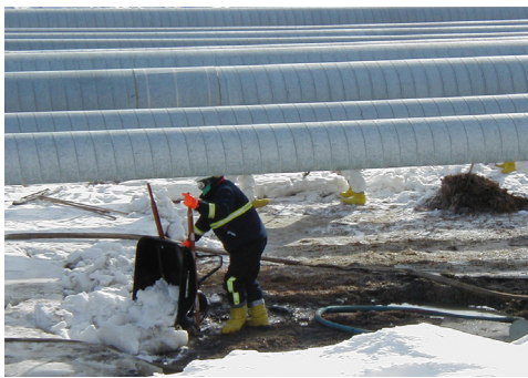
Figure 21. Using snow as a sorbent
