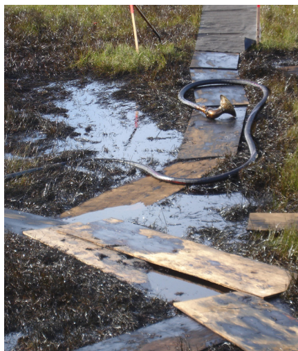
Figure 38. Vacuum hose recovering oil from low spot
