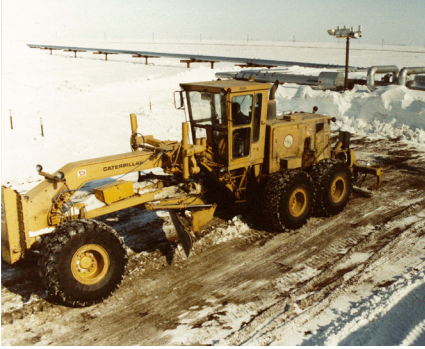
Figure 56. Scraping soil saturated with oil
