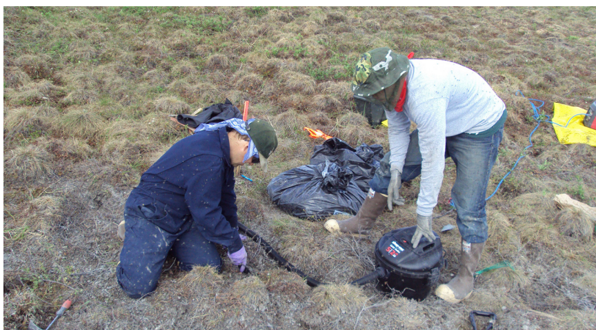
Figure 24. Vacuuming drilling mud
