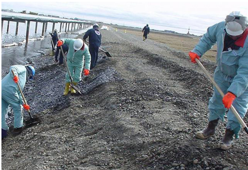
Figure 22. Shoveling contaminated gravel
