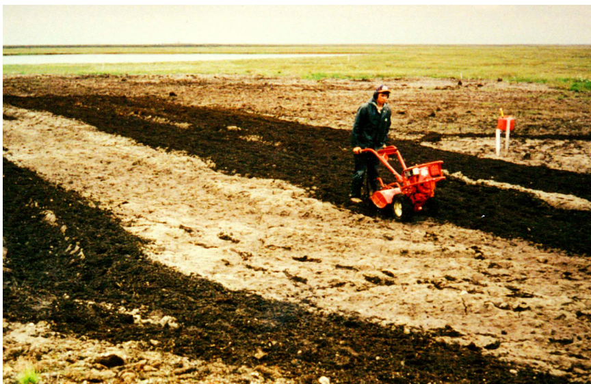
Figure 86. Rototilling contaminated soil
