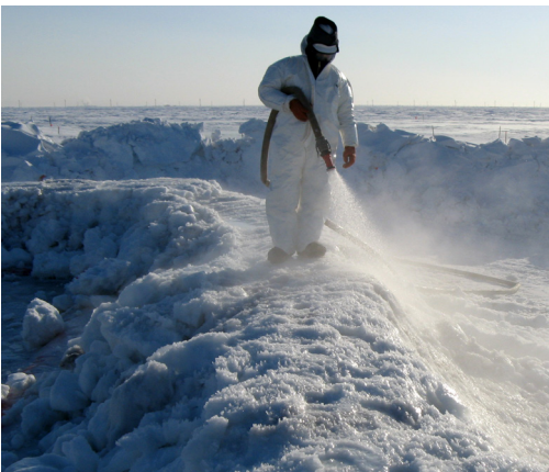
Figure 34. Constructing a snow and ice berm
