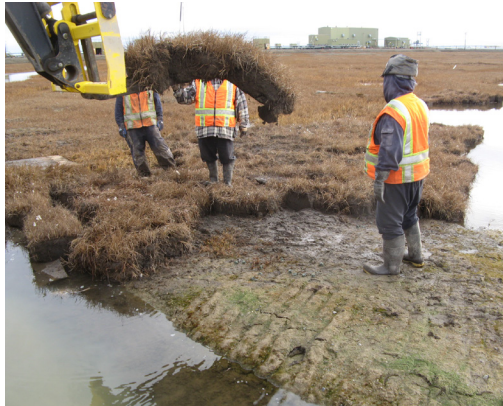
Figure 112. Moving large sod pieces
