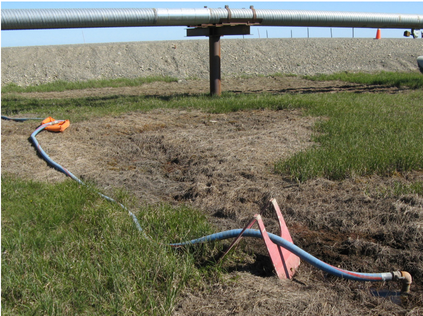
Figure 85. Dewatering to aerate soil
