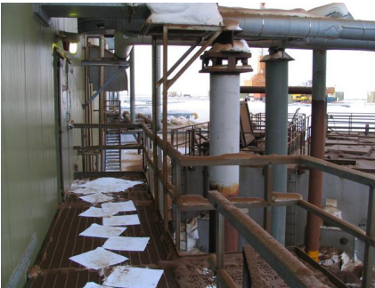
Figure 19. Sorbent used to prevent spread of contaminants
