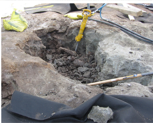
Figure 67. Excavating frozen soil with jackhammer
