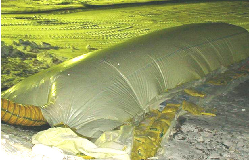
Figure 76. Heated tent to thaw soil
