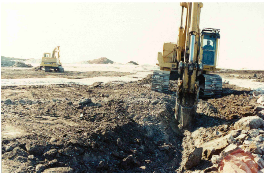
Figure 64. Backhoe excavating contaminated soil
