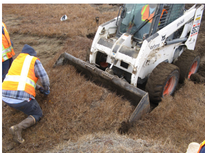
Figure 108. Harvesting sod with a small loader
