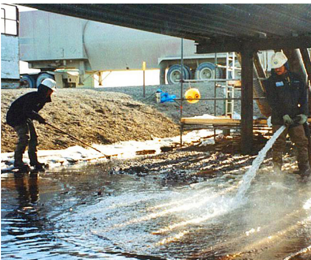
Figure 46. Flushing ice to mobilize oil
