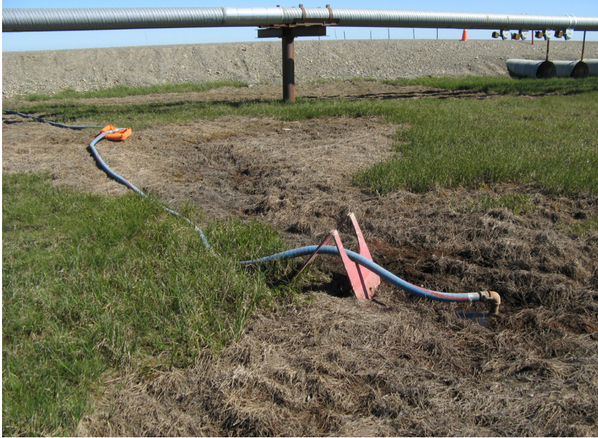
Figure 70. Natural low spot used for dewatering
