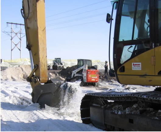
Figure 49. Excavating trench in ice
