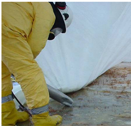
Figure 23. Vacuuming liquid contaminant
