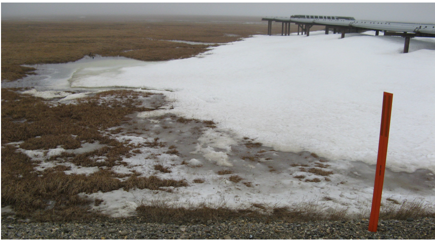
Figure 75. Snow drift on site not protected by snow fencing
