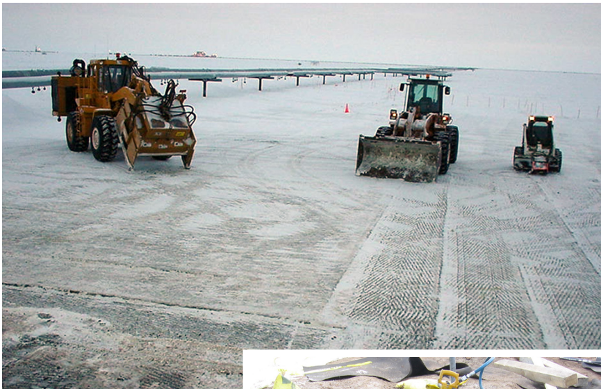
Figure 66. Site after excavation with trimmer
