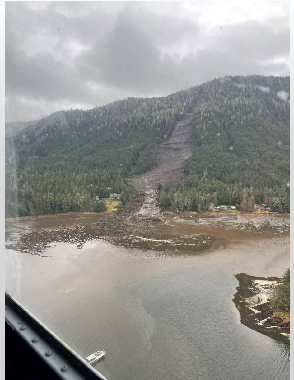
Wrangell Landslide as seen from CG-6026 on November 18, 2023
