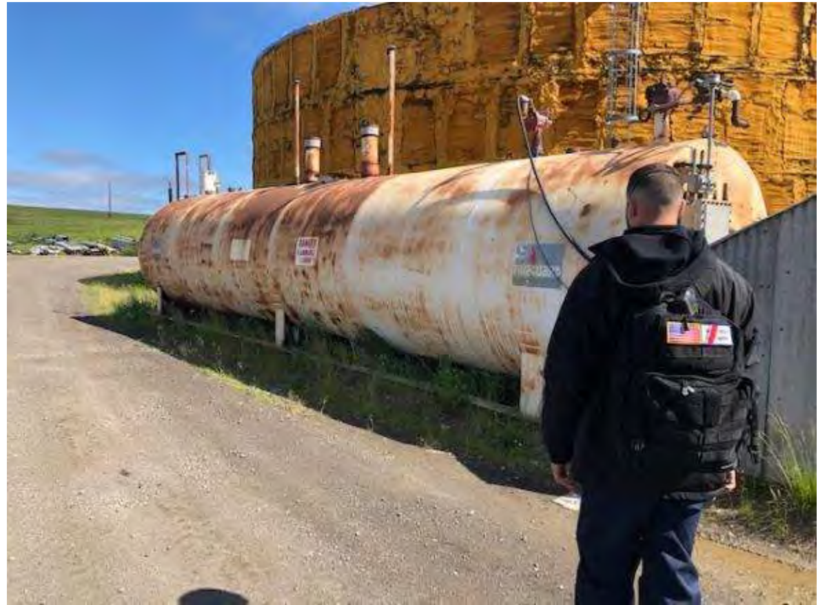
July 2020: Facility Inspection, Nome, AK
