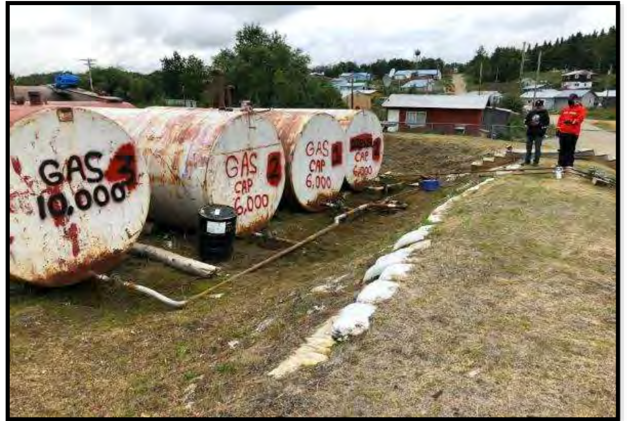
July 2020: Facility Inspection, Mountain Village, AK
