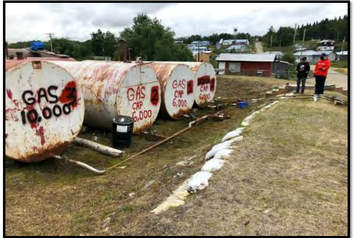
July 2020: Facility Inspection, Mountain Village, AK
