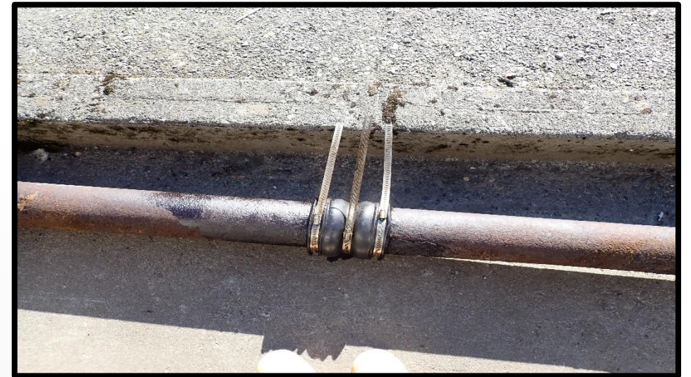
Corroded piping leak
