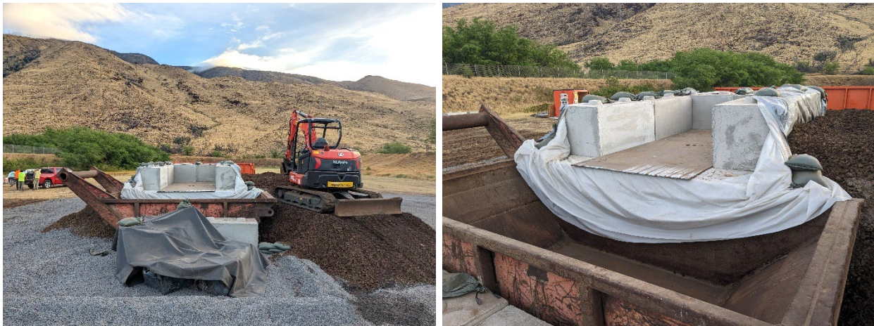
Figure 13: Battery termination setup where batteries are first processed to determine if de-energizing is necessary.
