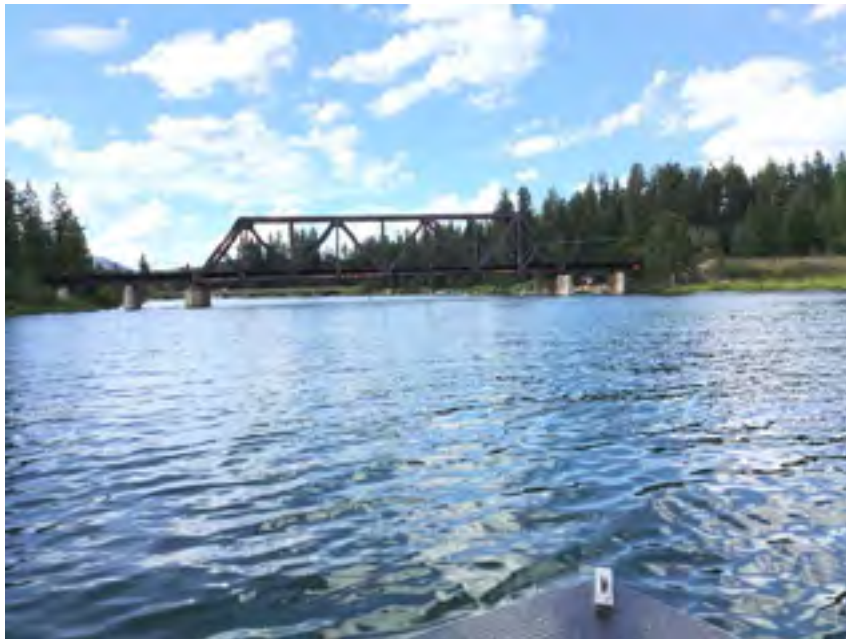
Looking at the staging area from the east
