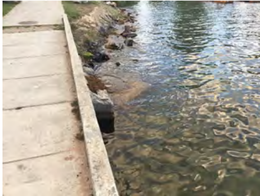
Image of concrete submerged culvert.
