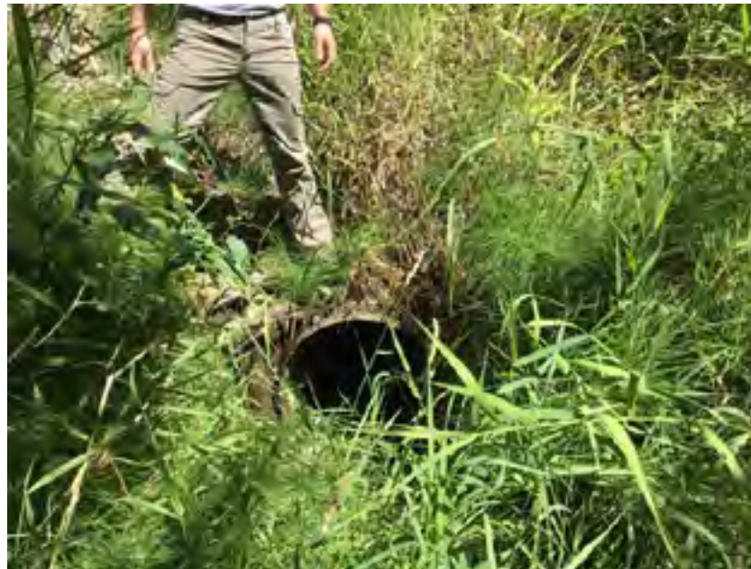
Facing east directly in front of culvert.
