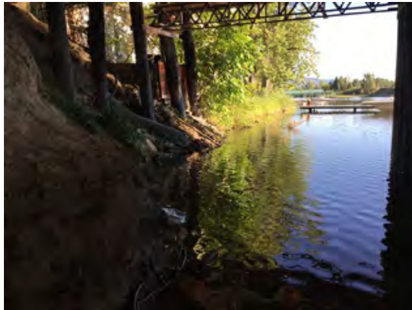
View from south of both culverts facing north.
