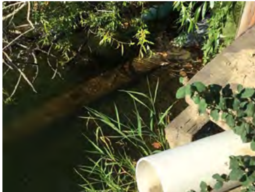
View from north of culverts facing south.
