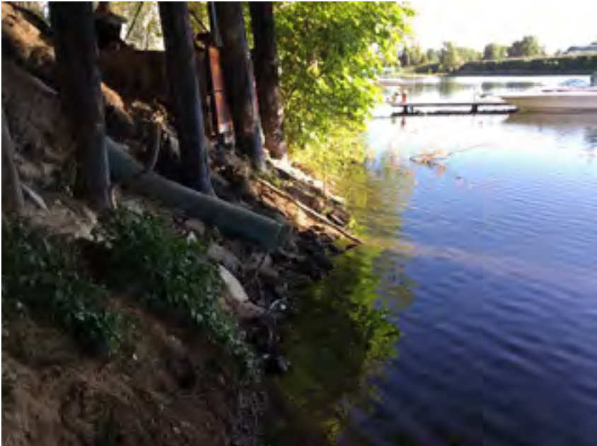
Image of concrete submerged culvert.
