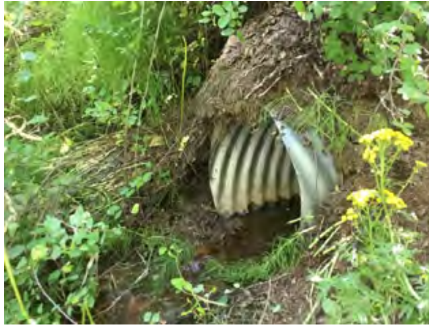
24 inch metal pipe culvert below gazebo, 15+ ft from shore.
