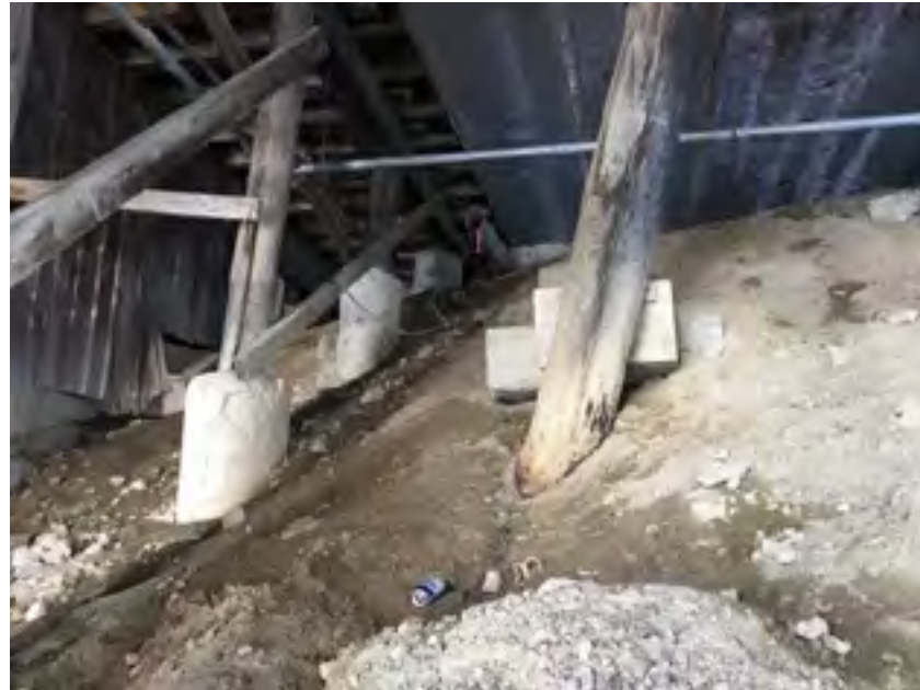
View of the southern culvert under bridge/restaurant.
