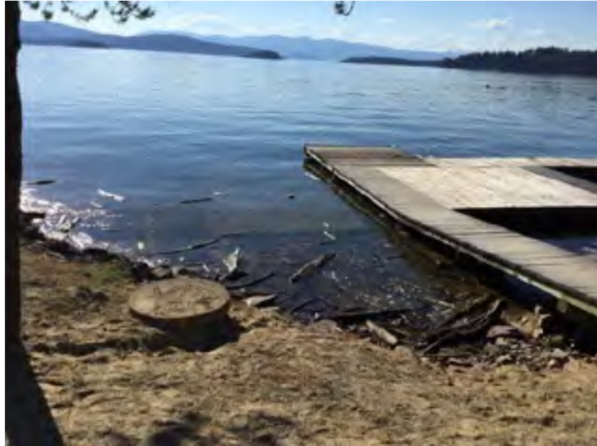
Surface water intake.
