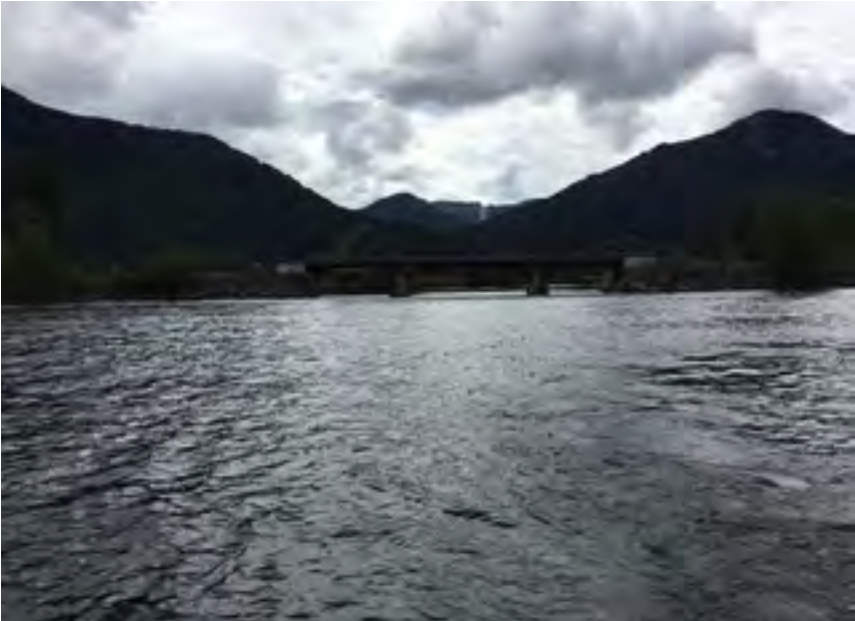
Looking South, towards Johnson Creek road bridge over Clark Fork South braid.
