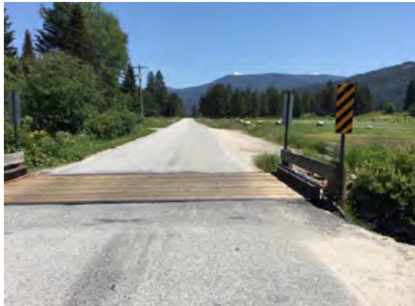
Looking east across bridge at parking area.
