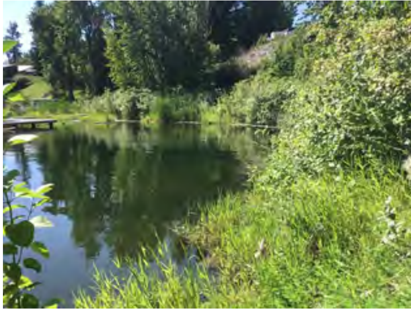
Looking Southwest towards outflow area of culvert, closer view.
