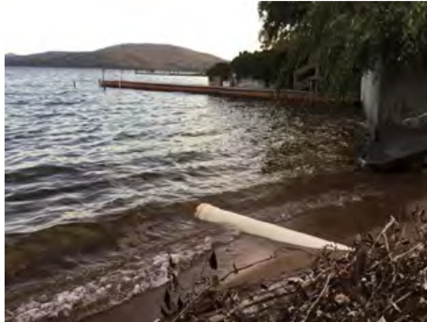
View looking south from north of culvert.
