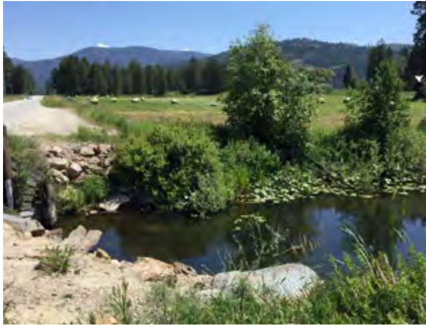
Upstream side of bridge showing creek and culvert.
