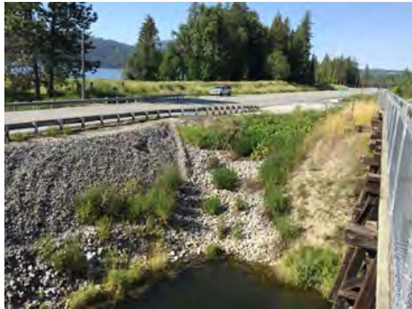
Small pullout on west side of bridge.
