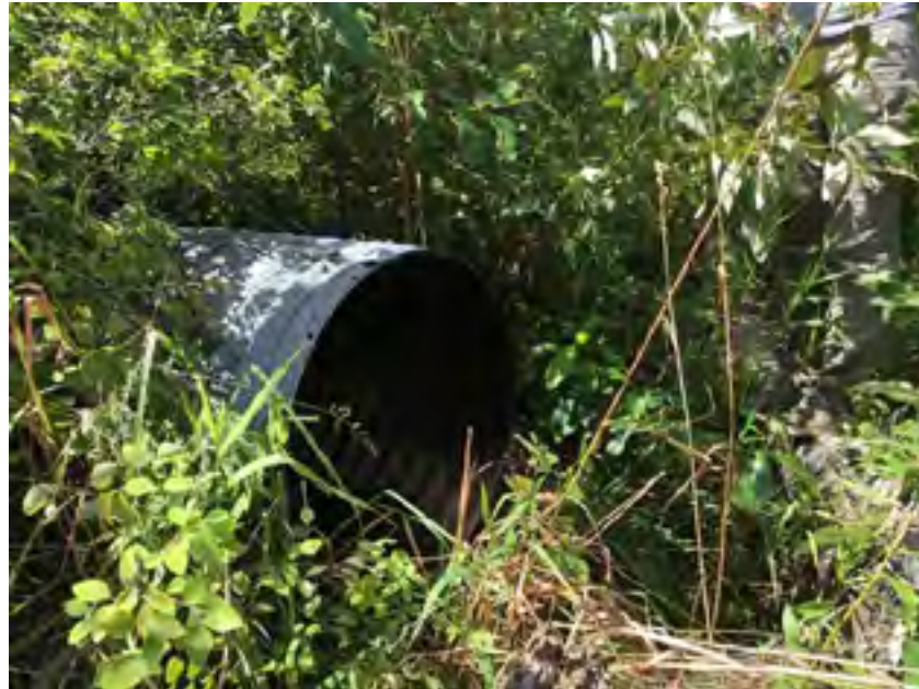
14 inch culvert South of railroad trestle.
