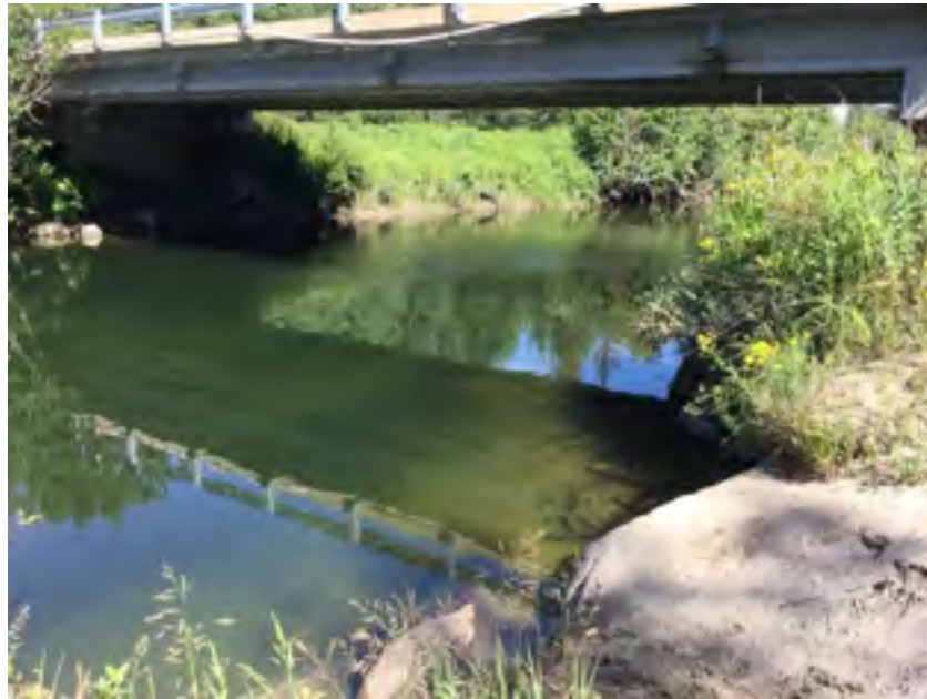
Looking north from collection point on River right to upstream anchor on River left.
