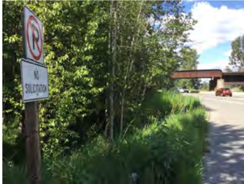
From turn off facing north with sign for orientation, culvert is central in frame.
