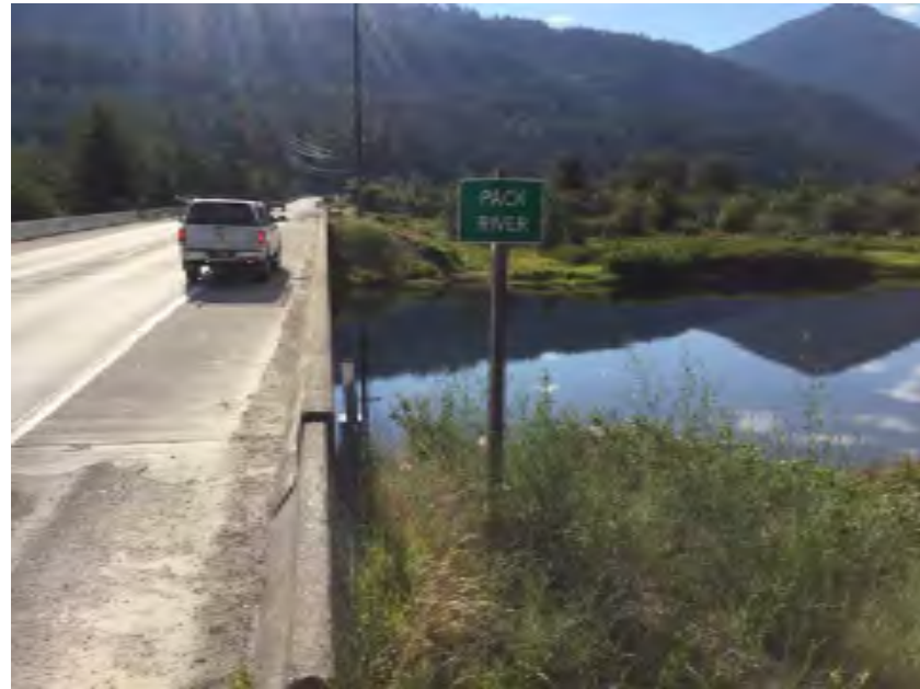
Pack River bridge from SR200 east bound.
