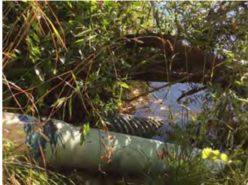
View from south facing north.
