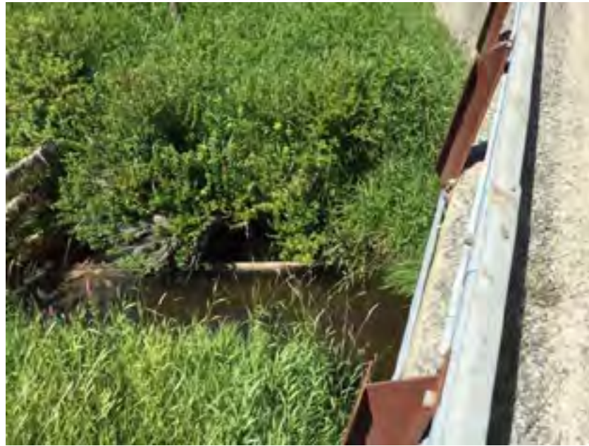
Looking west at the upstream end of culvert and strategy area.
