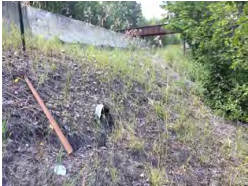
24 culvert South of railroad trestle, just below and downstream of 14 inch culvert.
