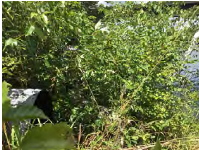
Picture of culvert facing downriver.
