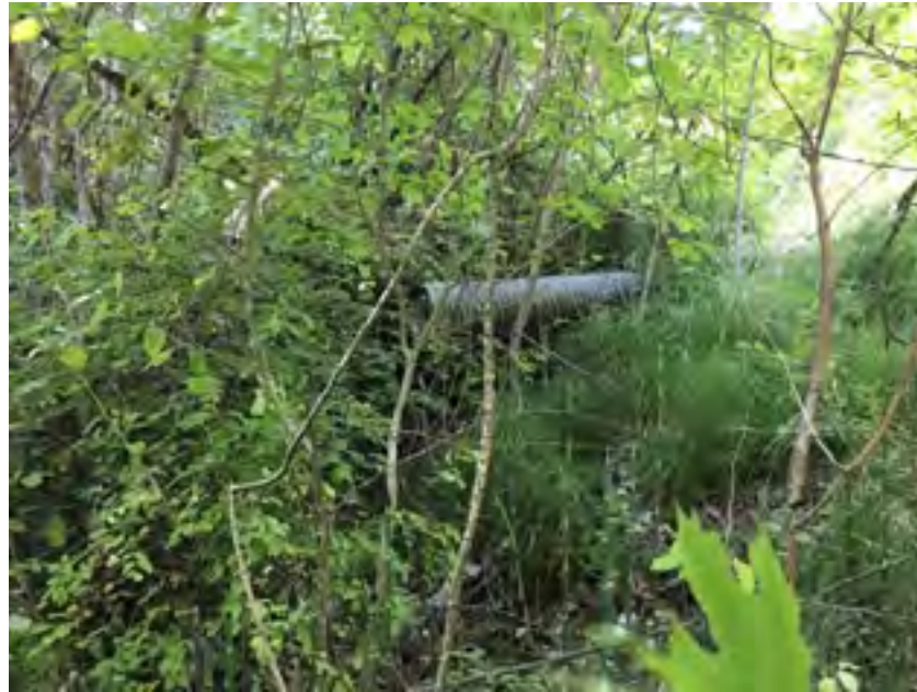
Smaller metal pipe culvert, closer to parking lot.
