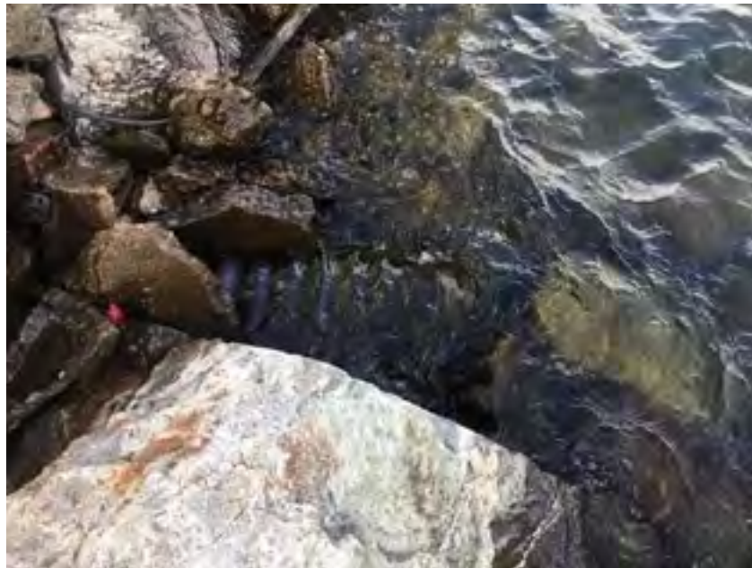
View of culvert.
