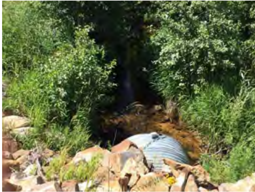
Looking south at upstream end of culvert and collection point.
