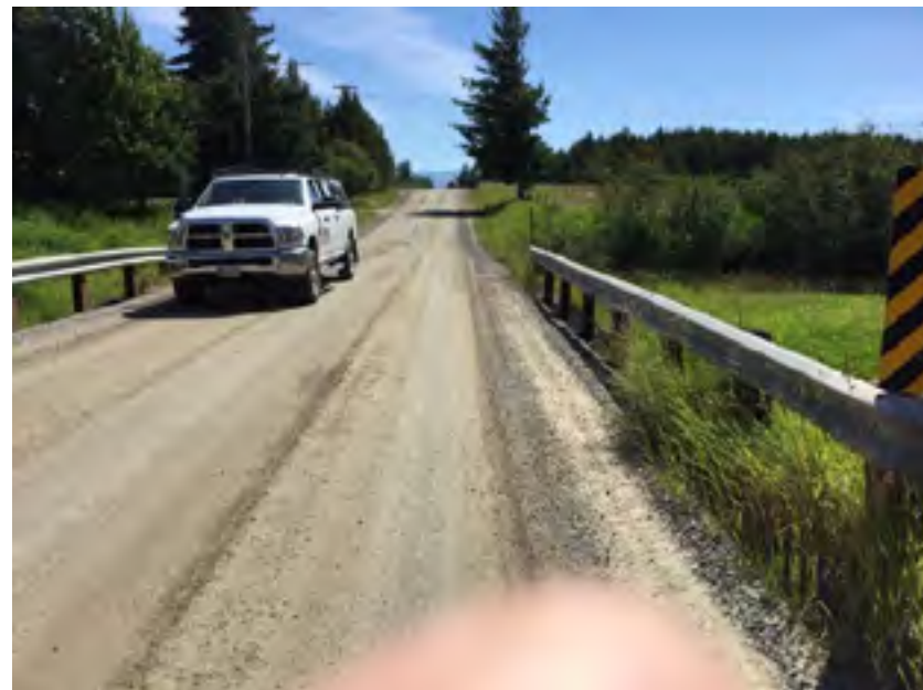
Looking east across bridge.
