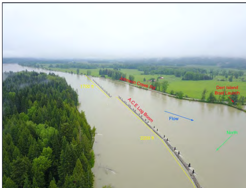
Looking downstream, where the most upstream piece of boom would be placed.
