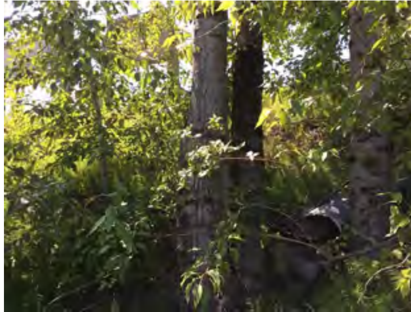
14 inch diameter metal pipe culvert, roughly 10+ ft from shoreline.
