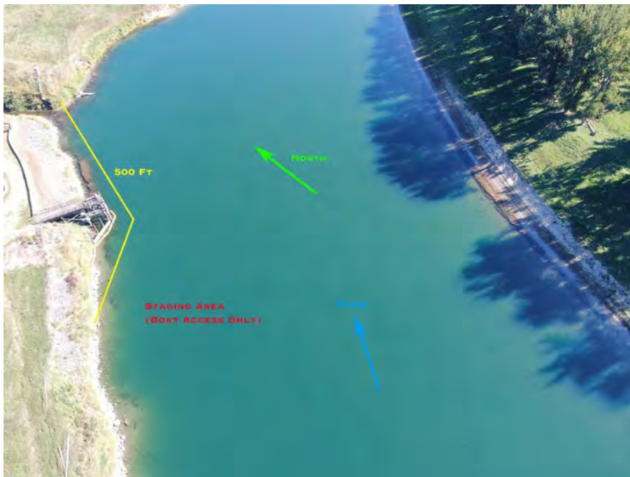
View looking downstream at Elk MTN Irrigation Intake
