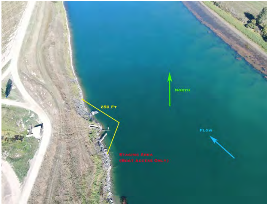
View looking downstream at Elk Mountain Farms Irrigation Intake
