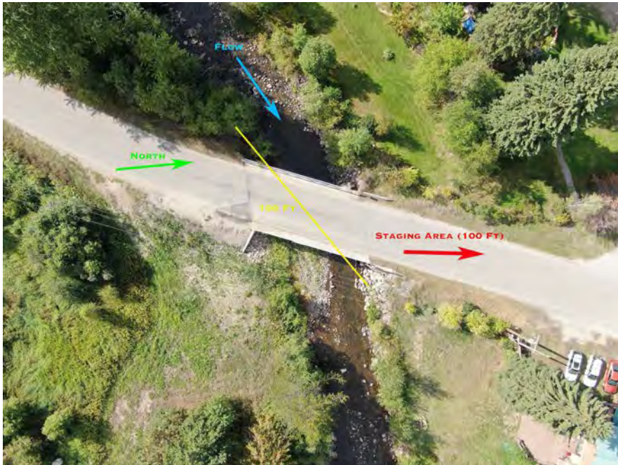
Overhead view of Deep Creek Loop Bridge
