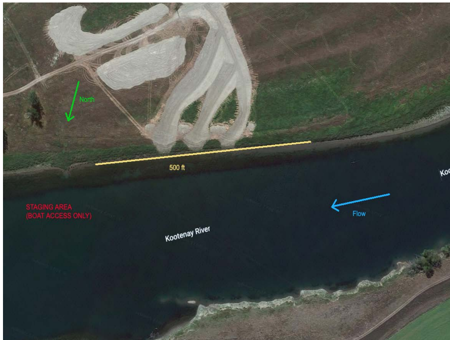
View looking from above Nimzs Ranch Intake 3
