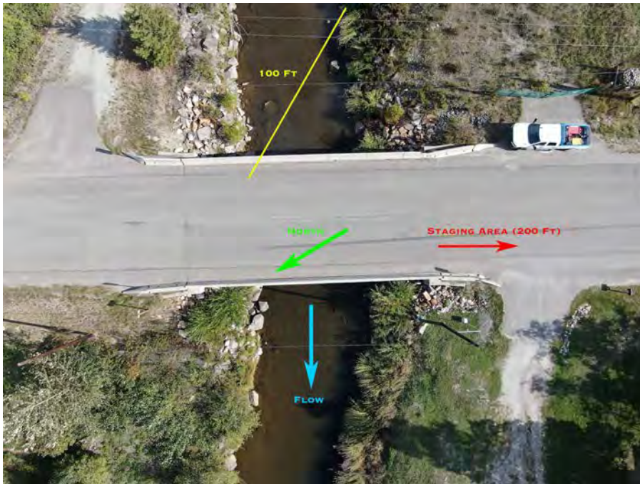
View looking upstream at South Boundary Fire Collection site.
