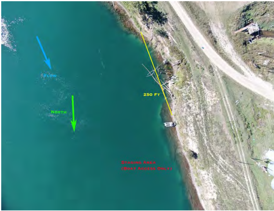
View looking upstream at Parker Creek Ranch Irrigation Intake
