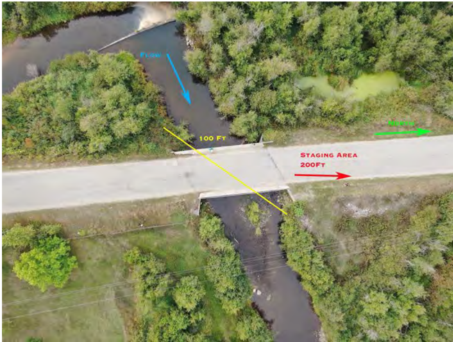
Overhead view of Deep Creek Campground Bridge
