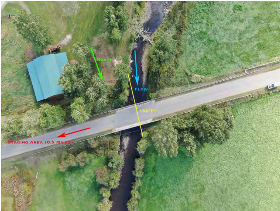
Overhead view of Lions Den Road Bridge
