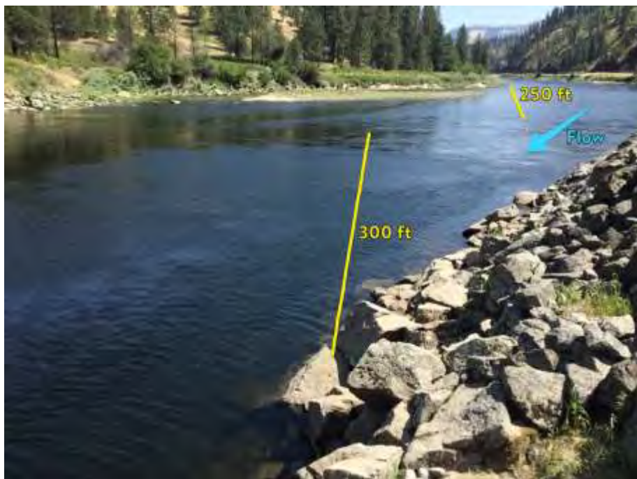
Looking upstream from collection site towards midstream anchor and upstream deflection.
