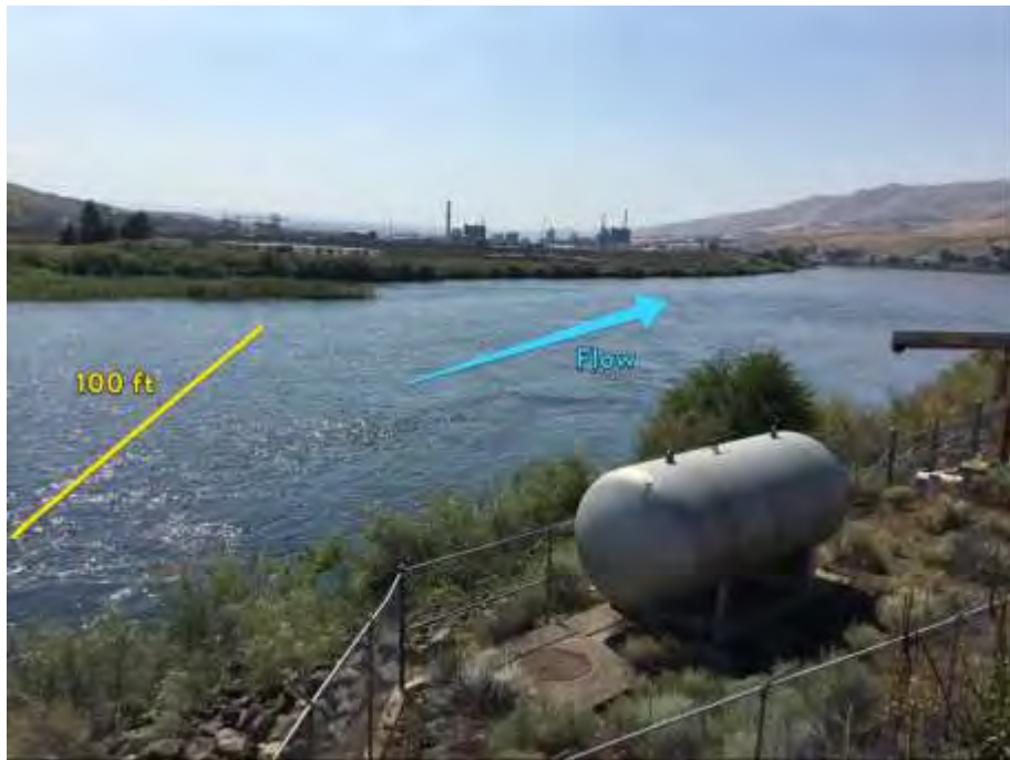
Looking downstream at exclusion site for water intake
