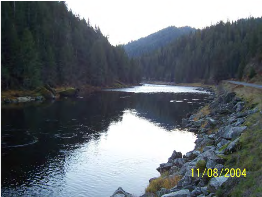
Shoreline Type 6C: Exposed rip-rap.
