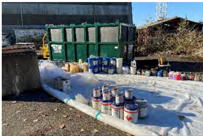
Miscellaneous HAZMAT removed
