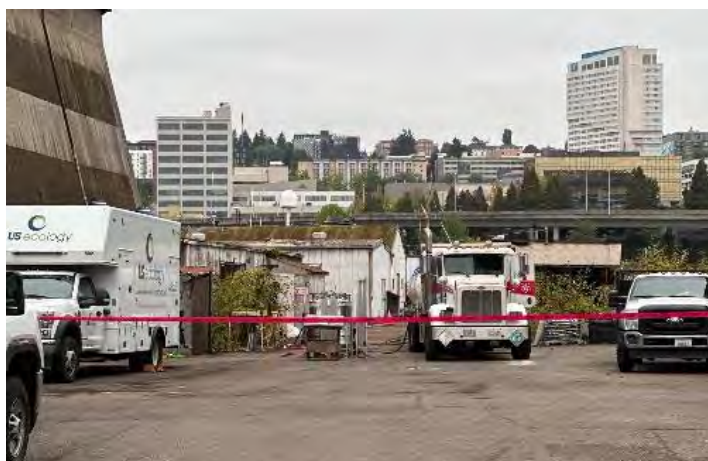
Vac Trucks removing Anhydrous Ammonia
