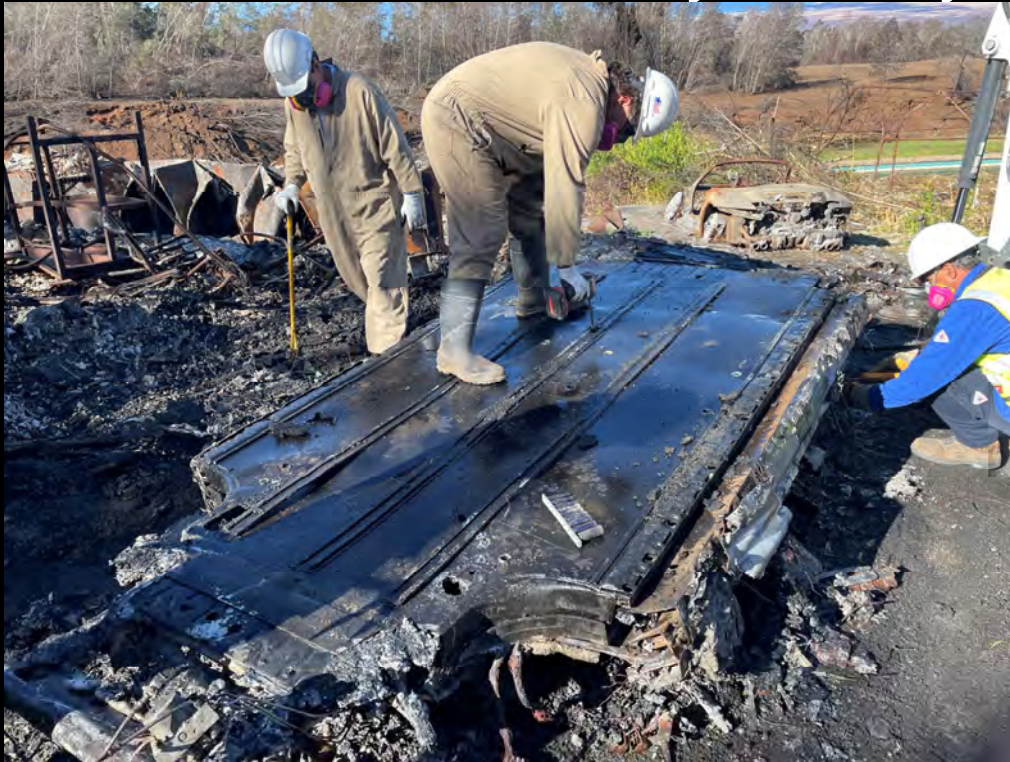
Step 3: Remove Fasteners & Central Strip
