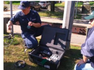
(Above) PO2 Josh Rice and EPA Region I START Contractor set-up Air Monitoring Unit in Wellesley, MA
